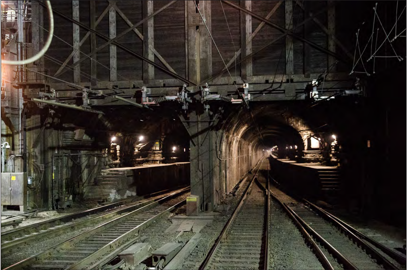
Entrance to the North River Tunnel in New York
