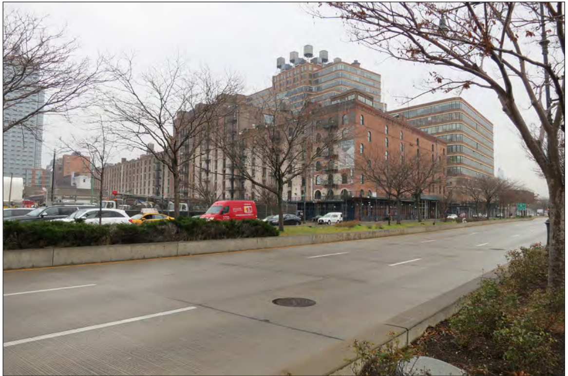
View southeast on Twelfth Avenue/Route 9A of the New York Terminal Warehouse Company buildings 16 and the Starrett-Lehigh Building south of it in the West Chelsea Historic District.
