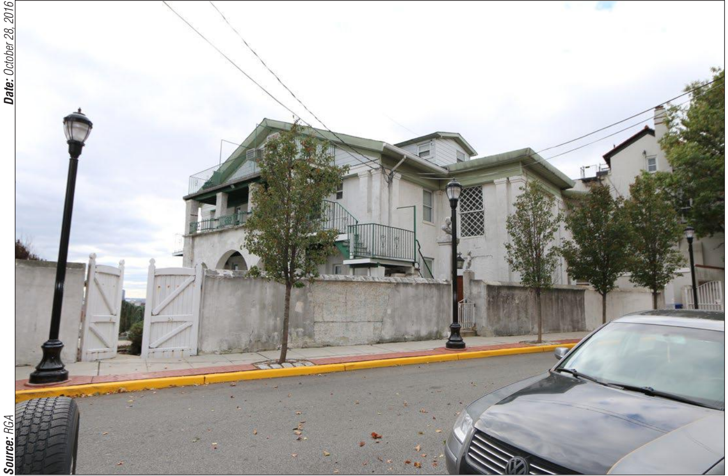
View southwest of 320-324 Mountain Road, north and east elevations, in the City of Union City. 10
