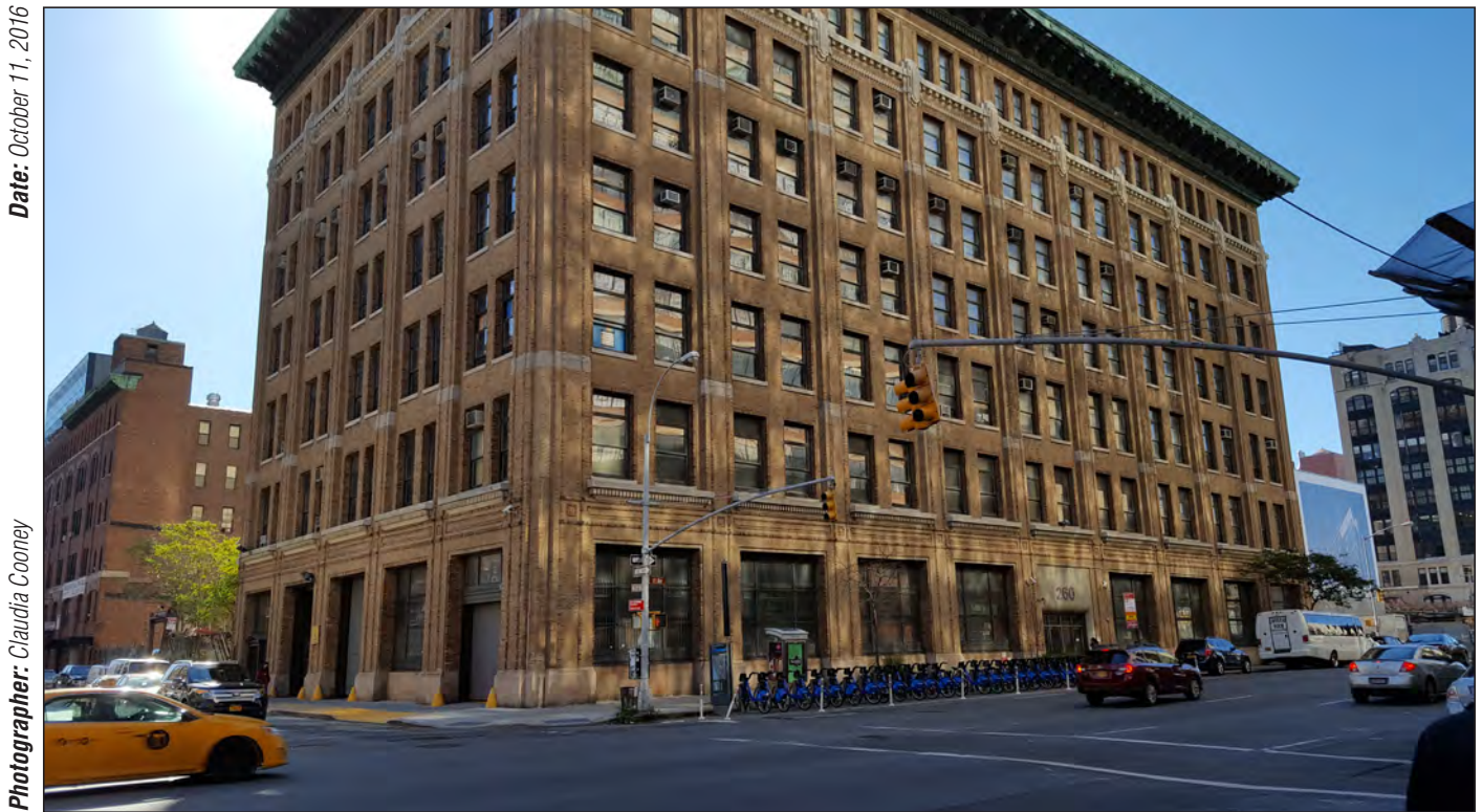
Otis Elevator Building in West Chelsea Historic District, 246-260 Eleventh Avenue. View southeast on Eleventh Avenue. 14
