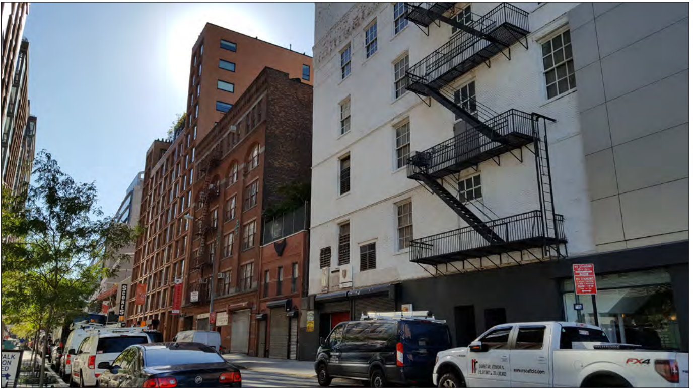
View of the south side of West 28th Street, east of Eleventh Avenue, 17 in the West Chelsea Historic District.
