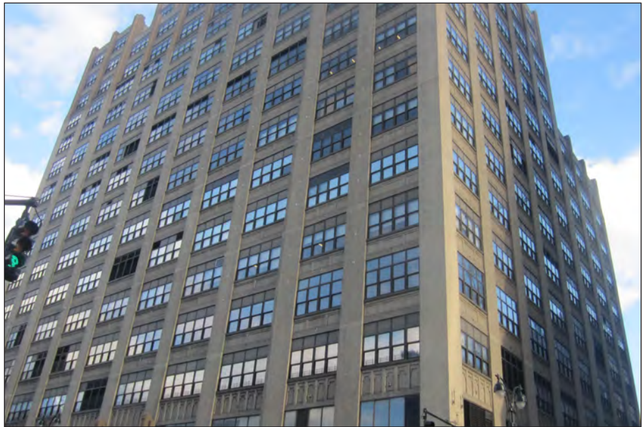
Master Printers Building, 406-416 Tenth Avenue. View northeast from Tenth Avenue and West 33rd Street.
